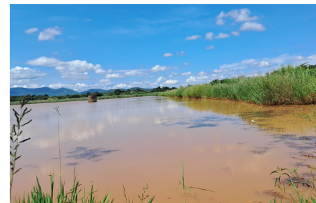
EWSC'S LUTEMBWE DAM 1 WITH HIGHLY TURBID WATER
